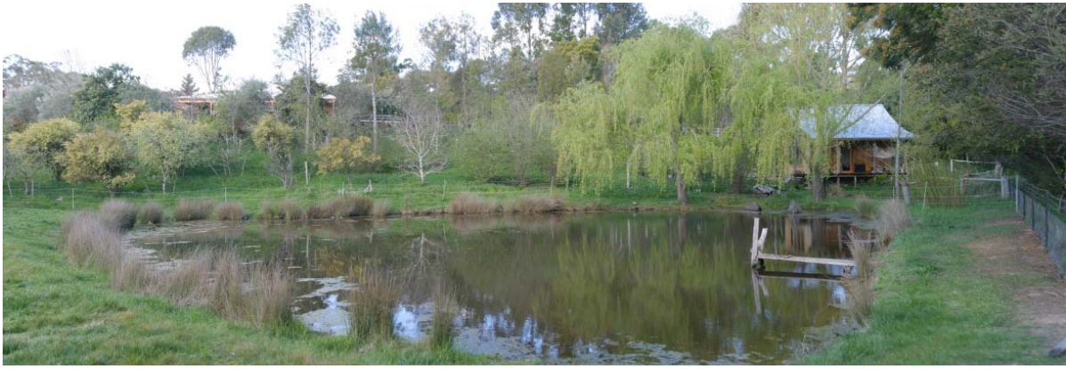
Figure 12 One megalitre dam collecting town stormwater runoff at Melliodora; a key element in maintaining an extensive irrigated orchard and providing fire fighting capacity (including additional source for CFA tankers)
