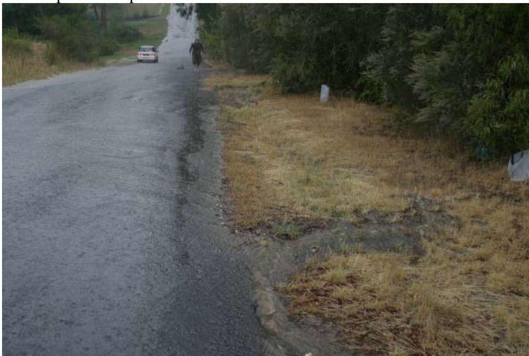
Figure 13 Small street side storm water diversion to contour swale 14 th St Hepburn
